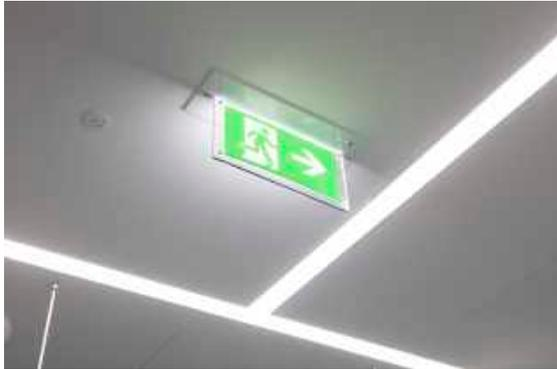
A unique feature of Lightmatrix is its ability to not only support any luminaire suppliers' fixtures, but also fully support emergency lighting. Working with our ICEL (Industry Committee for Emergency Lighting) approved partners LitePlan and ELP, we support self-contained emergency lighting for 3-hour emergency autonomous operation along with fully automated emergency testing and reporting over PoE. This significantly reduced the cabling demand and allowed the delivery of a unified system.
