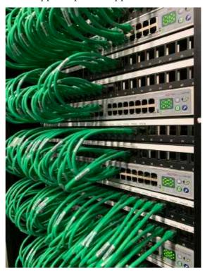
Our in -house design team scheduled all data cabling to ensure optimum loading and our engineering team worked closely with Bancroft's cabling provider TCG to deliver a clear and traceable patching architecture. The resulting installation is both simpler to manage and is modular for future changes.
